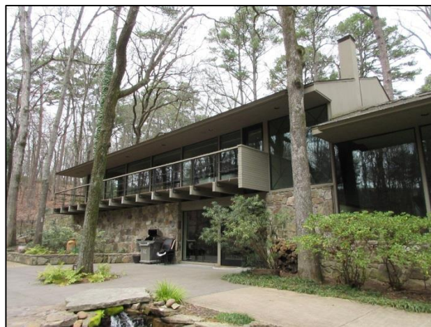
Rear elevation of Tiller House, 2016
